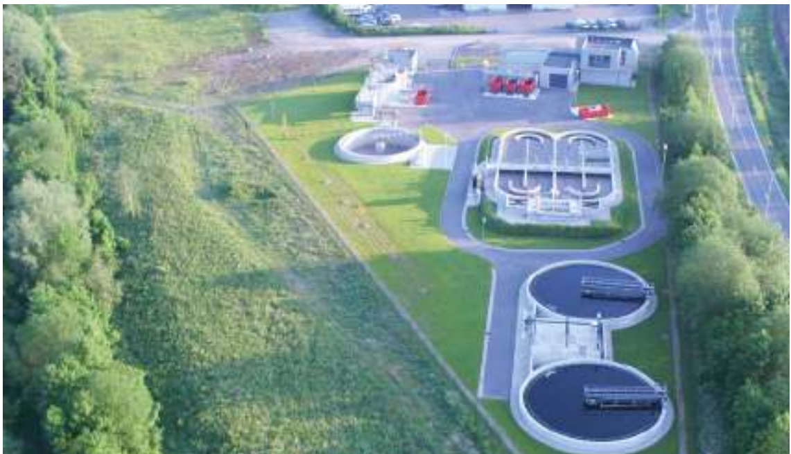
Godinne // Station d'épuration
