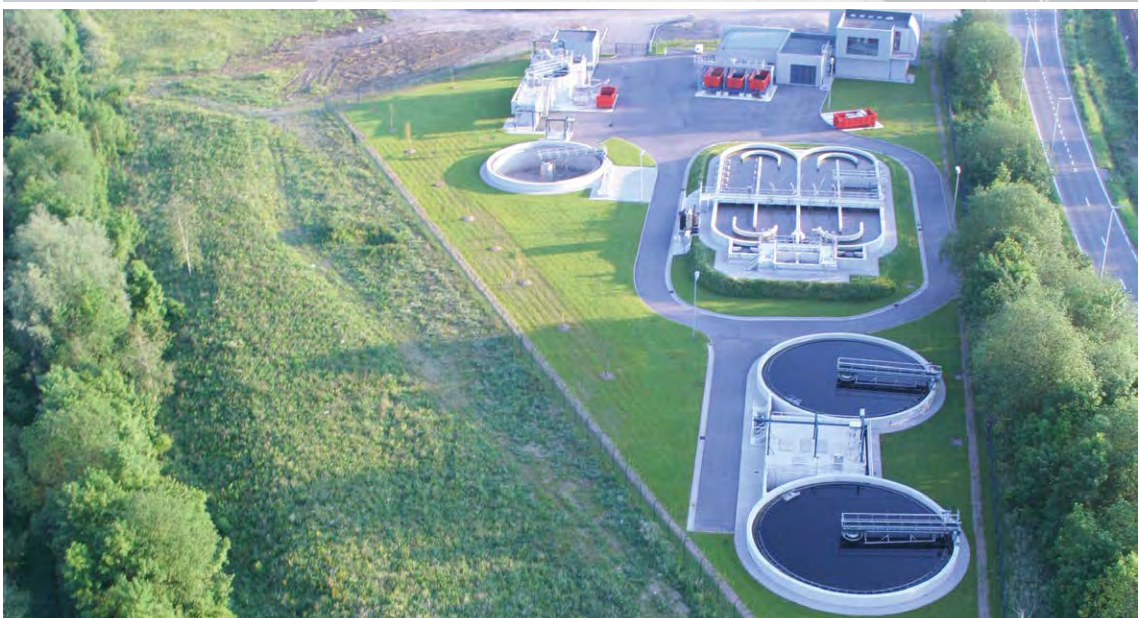
Godinne // Station d'épuration
